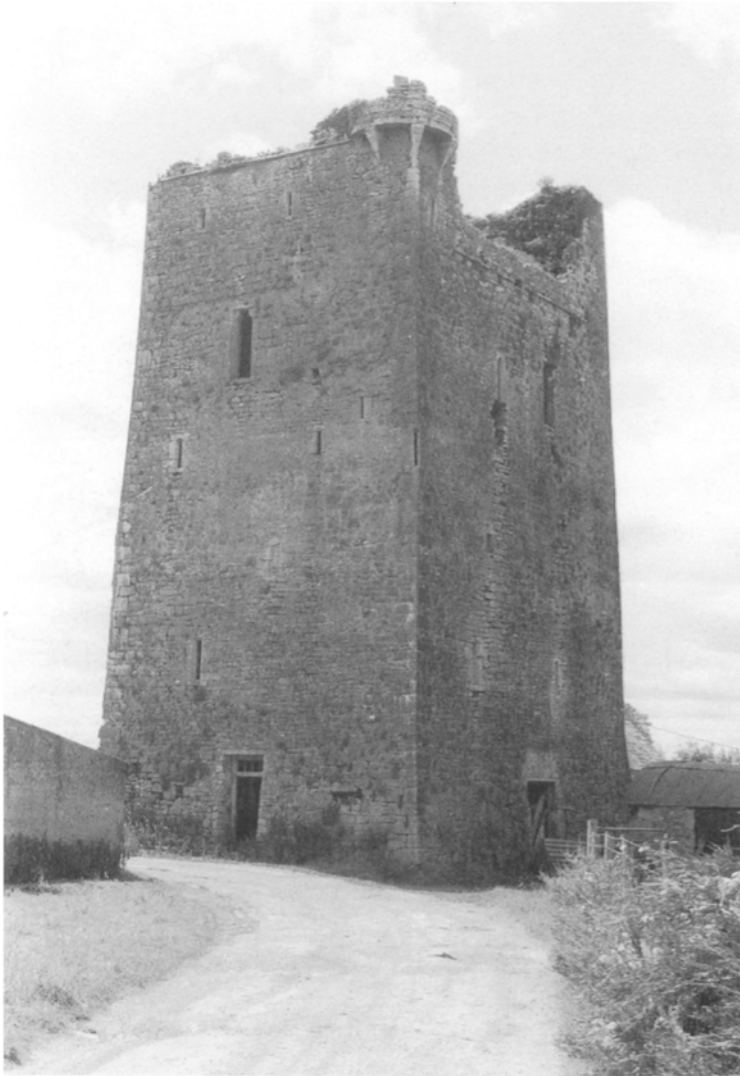
Figure 132 Two Mile Borris, Co. Tipperary: a Minister tower-house, without turrets but with machicolated corner turret
