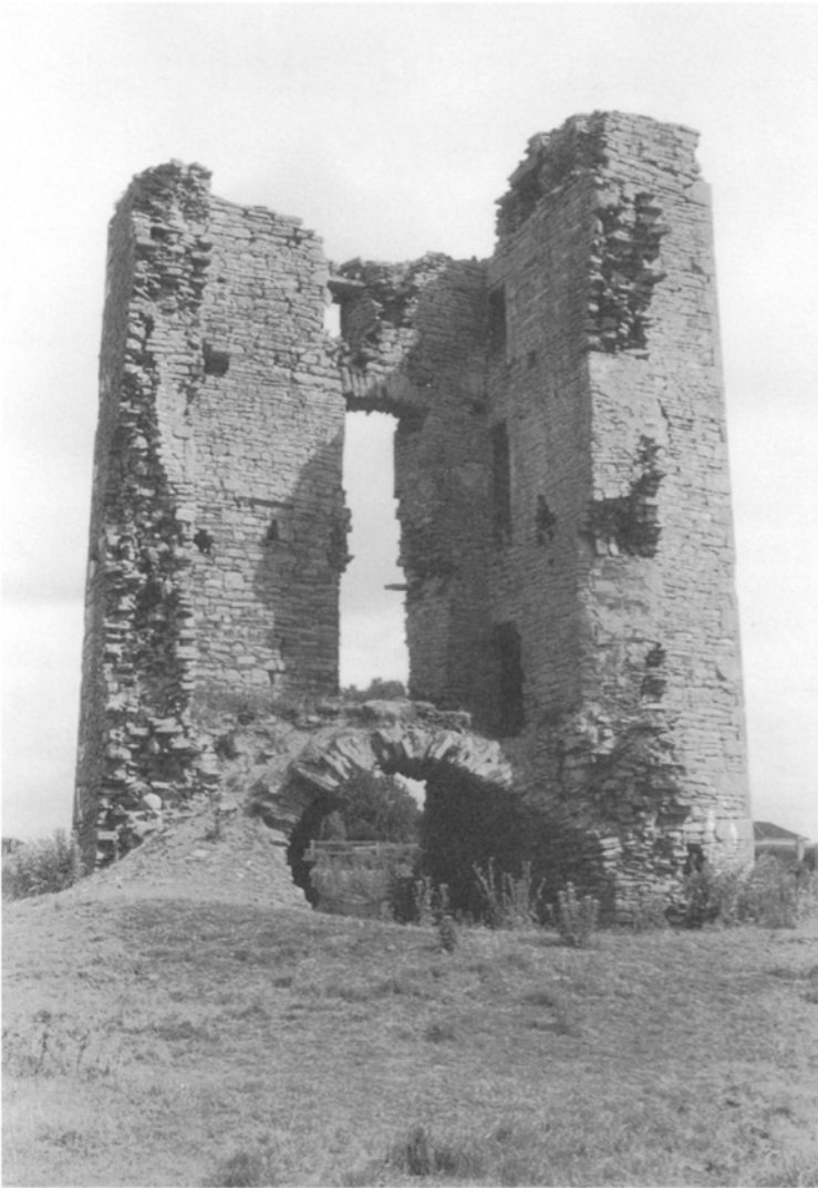
Figure 127 Walterstown, Co. Meath: the tower-house, showing the vault and floor levels
