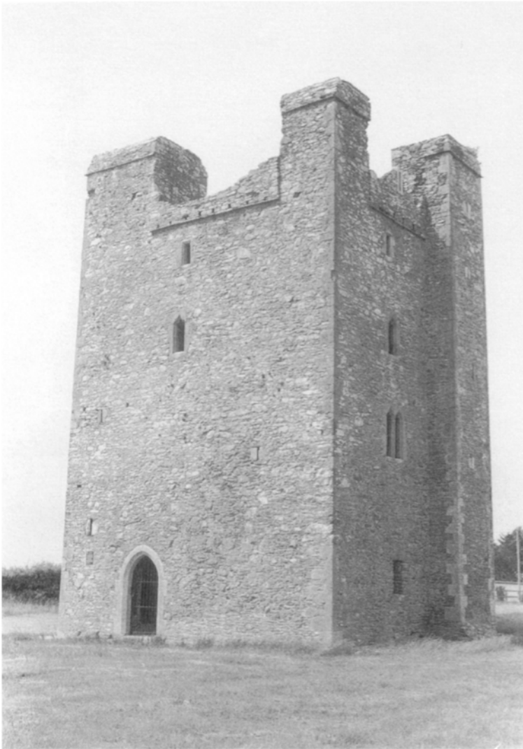
Figure 129 Roodstown, Co. Louth: the flanking turret does not protect the door of the tower-house
